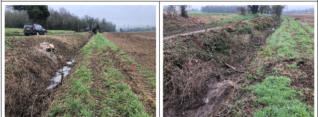
Figure 2 – Layby 2 vegetation clearance completed
