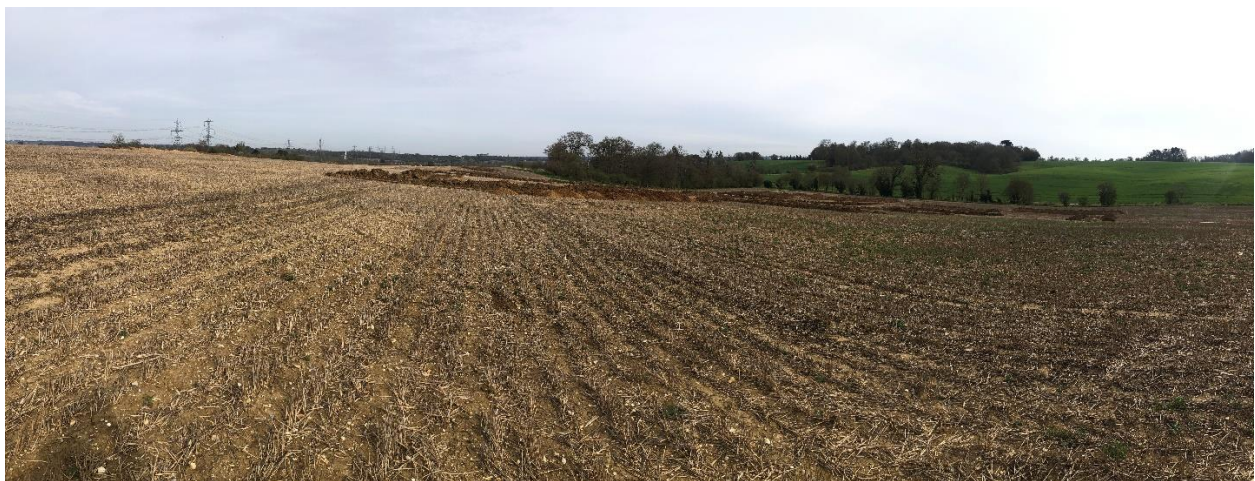
Figure 2 – Progress East of the EA cables and South of the Gas lines
