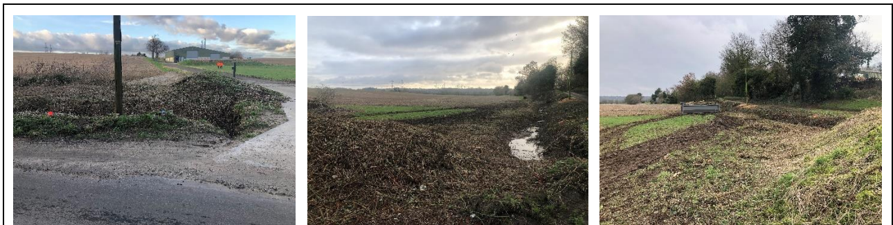
Figure 1 – Site entrance vegetation clearance completed
