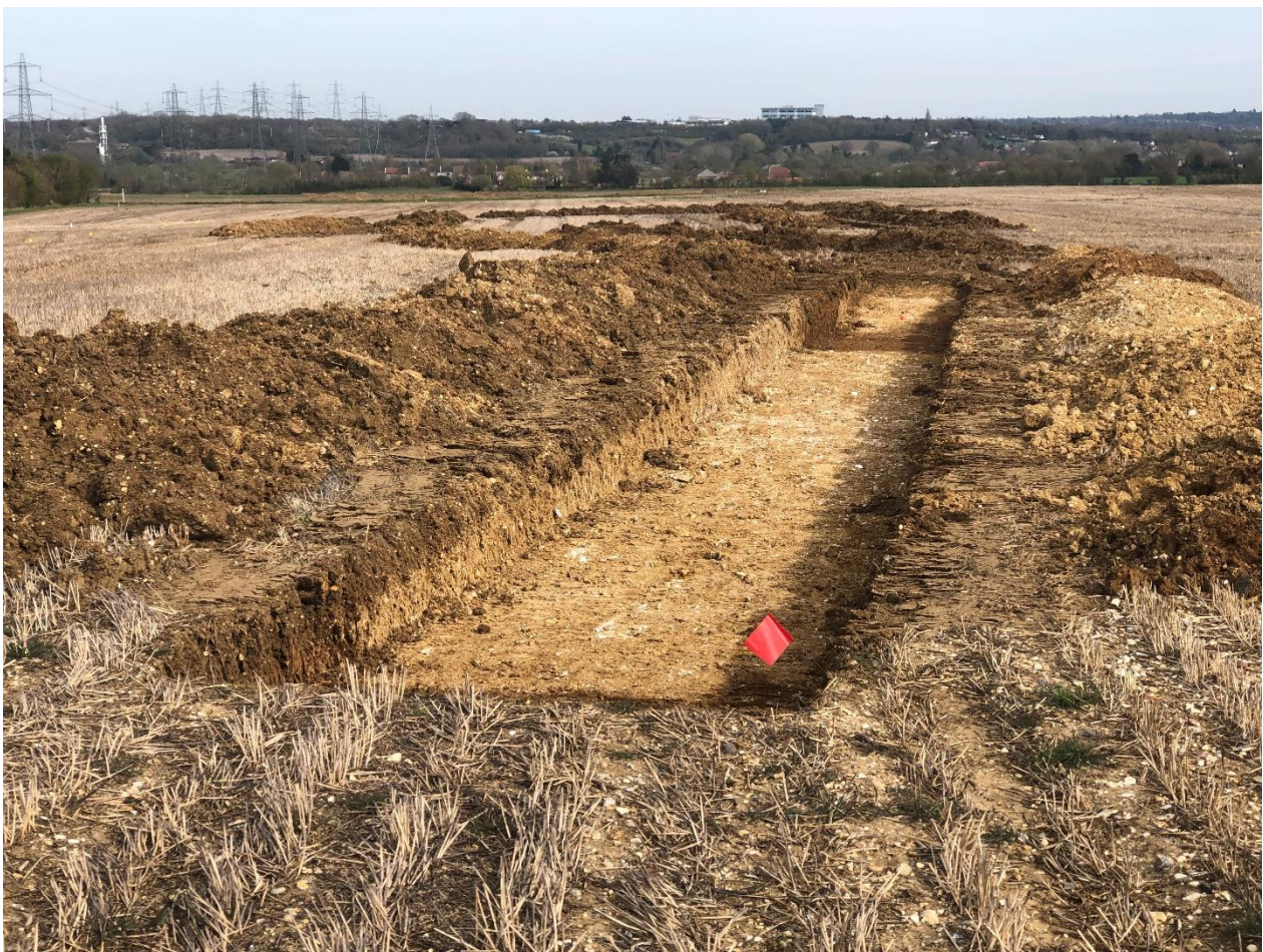
Figure 3 – Progress East of the EA cables and in-between the Gas lines
