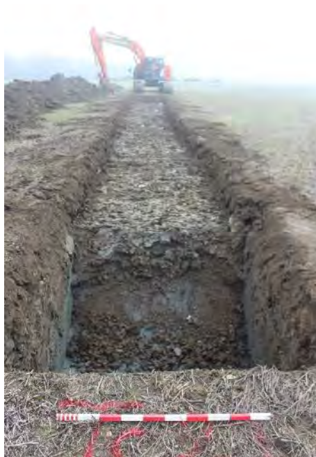
Trench 26, Facing East
