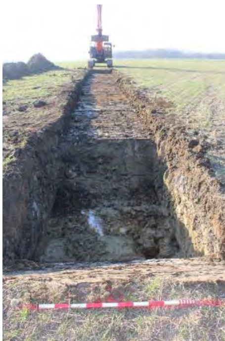
Trench 29, North Facing
