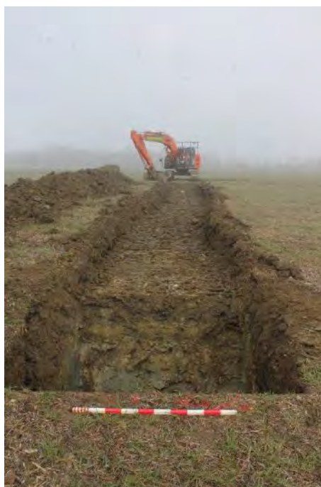
Trench 22, Facing West
