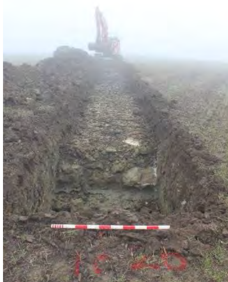
Trench 20, Facing West
